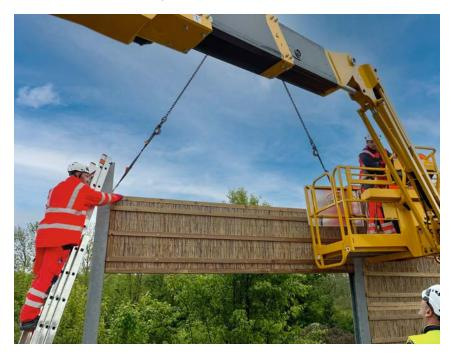
We are using the new noise protection reed wall to test the technical handling during construction, the noise-related effectiveness, its ability to resist the elements, and thus its service life and the effects during the operating phase. The result is a recommendation regarding whether building other such walls in the future.
